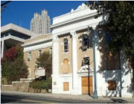
Atlanta Life Insurance building awaiting revitalization, Auburn Avenue
