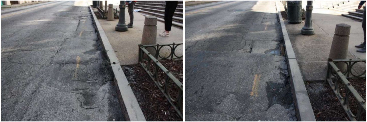
Figure 4.8 Pavement Warping Examples
