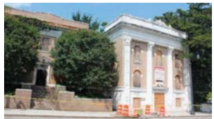
① Original Atlanta Life Building
